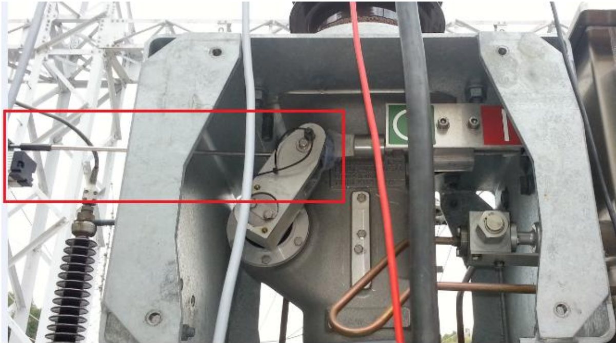
Figure 4. Linear transducer movable rod installed on movable part of CB
