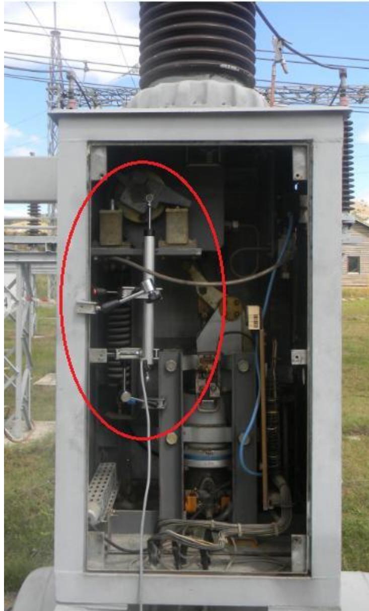
Figure 6. LWG linear (analog) transducer installed on Energoinvest SF6 123 kV CB, Type SFE 11/18-G
