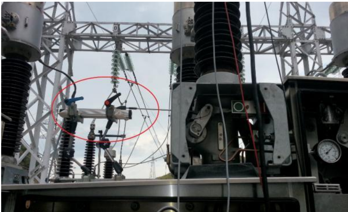
Figure 5. Linear (analog) transducer installed on Siemens 123 kV CB, Type 3AP1F
