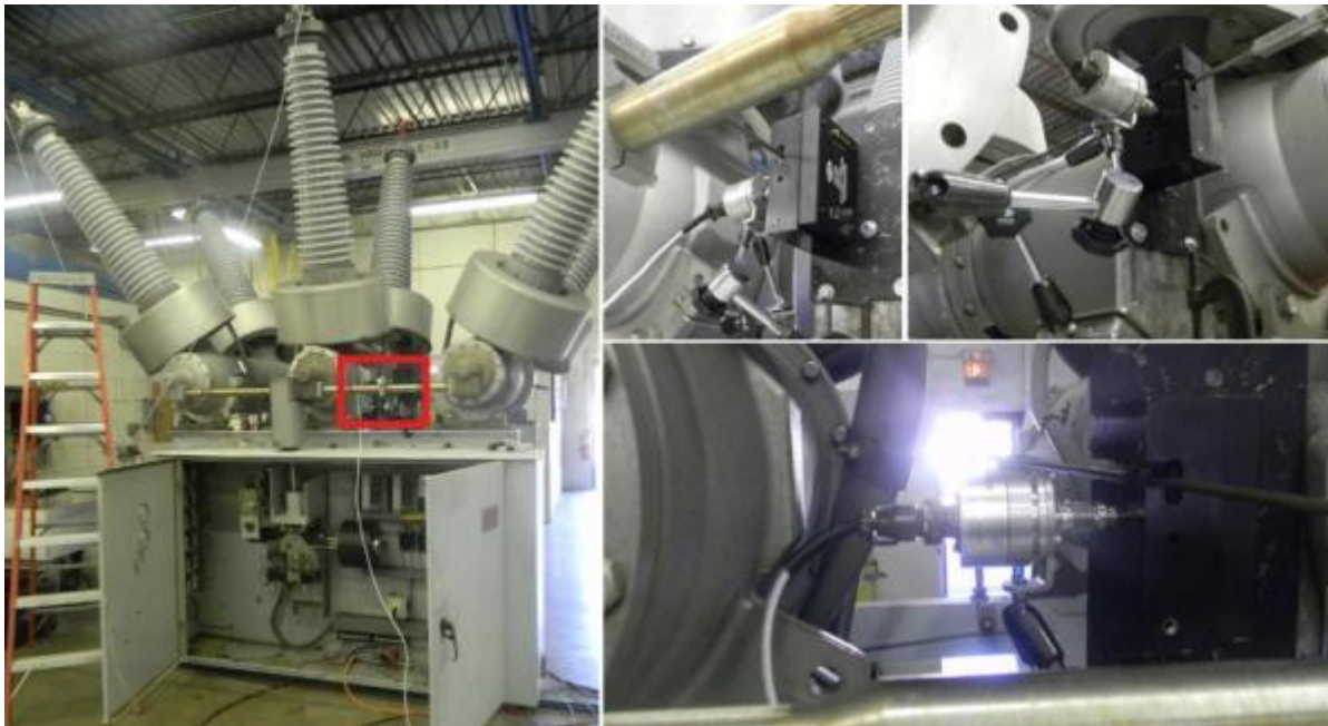
Figure 9. Rotary (digital) transducer installed on Dead Tank CB, ABB SF6 145 kV, Type 145 PM 63-20
